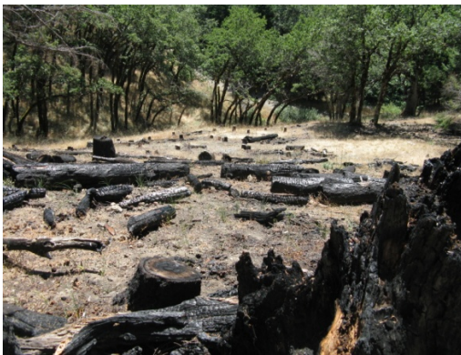
Cut and burned Douglas-fir, removed to defend a small prairie on Stormy Saddle Trail
